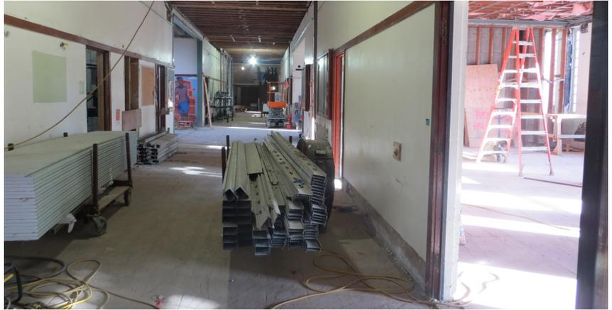
Area B2 seismic upgrades are wrapping up here soon. MEP/F system overhead rough-in is in progress with existing floor finishes in process. Interior wall framing is occurring on all floors. Fire rated ceiling metal framing followed by sheetrock is in process this month. The Area B2 Commons roofing is occurring this month followed along with installation of the MEP/F overhead rough-in. Many interior finish activities will begin to kick-off towards the end of this month.
